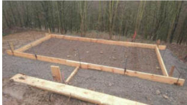
Abb. 4.13: Fundament Gasunterstation
